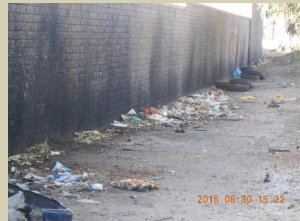
Figure 26 Various building are in serious need of repair and some properties have derelict building that are vandalised by criminal elements.
