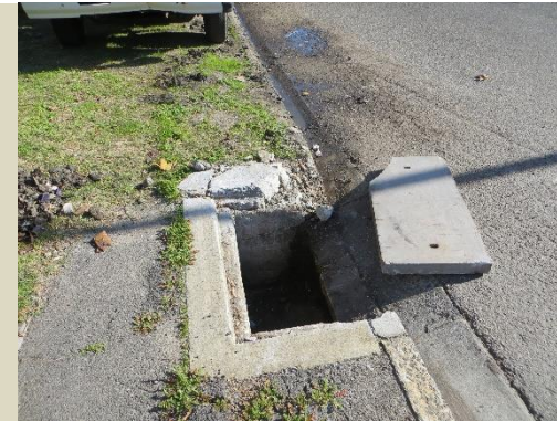
Figure 19 Broken manhole covers on sidewalks
