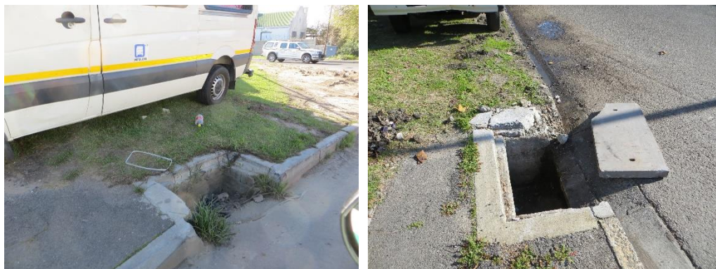
Figure 42 Storm water drains are blocked or completely absent due to poor road maintenance
