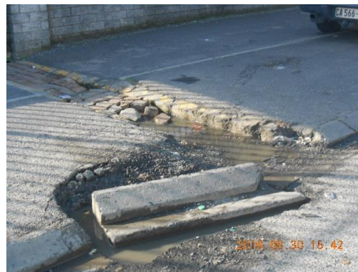
Figure 44 Some road surfaces, kerbs and gutters are badly maintained
